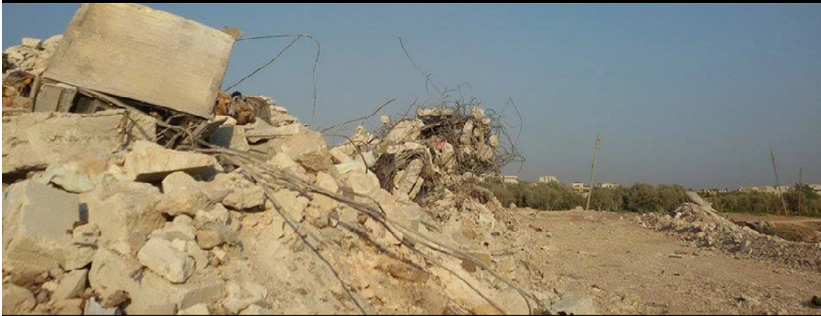
Image of the destruction of the 2 houses of Mou'awia Al Amouri from Attma village in Idlib country side due to International Coalition warplanes missiles, August 11, 2015
