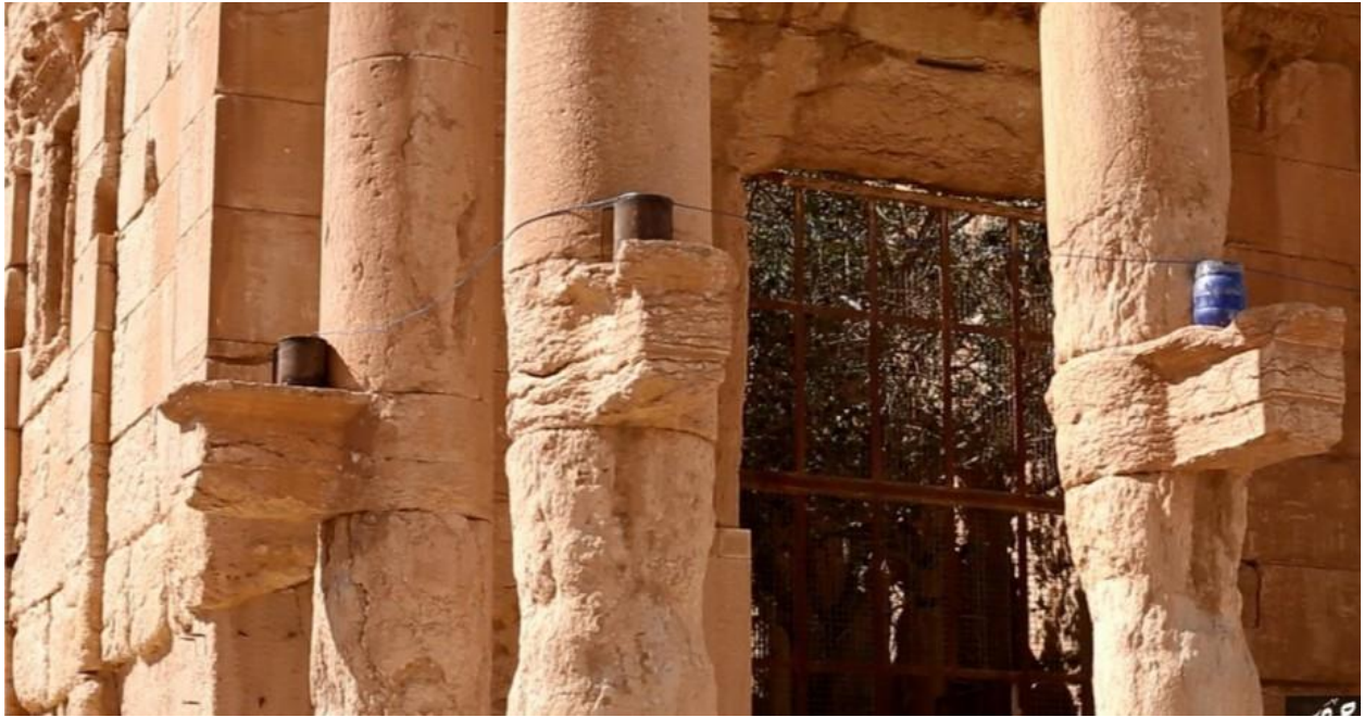
Baalshamin Temple, placement of explosives (APSA; August 23, 2015)
