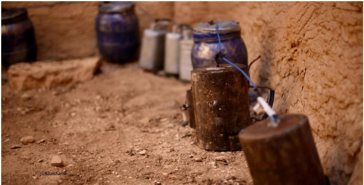
Baalshamin Temple, placement of explosives (APSA; August 23, 2015)
