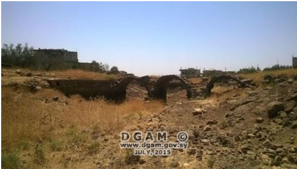
The Roman Bridge (DGAM; July 26, 2015)
