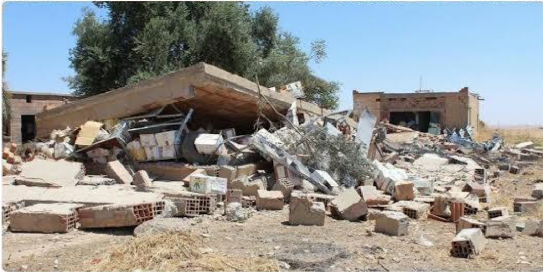
Tell Chuera Dig House, after damage (DGAM; July 26, 2015)
