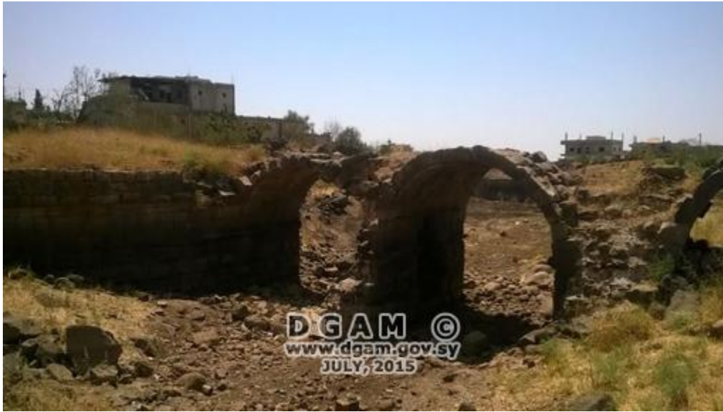
The Roman Bridge (DGAM; July 26, 2015)
