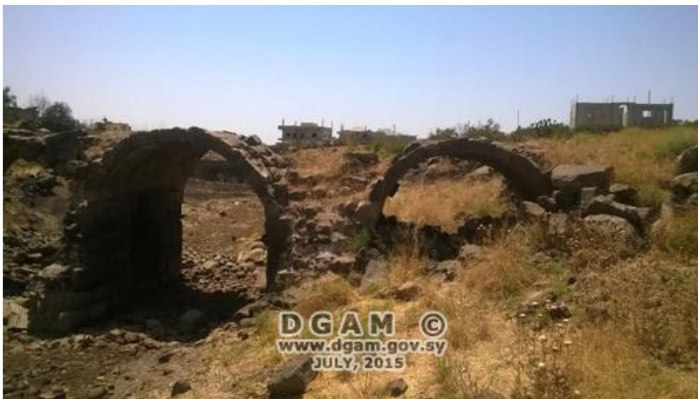
The Roman Bridge (DGAM; July 26, 2015)
