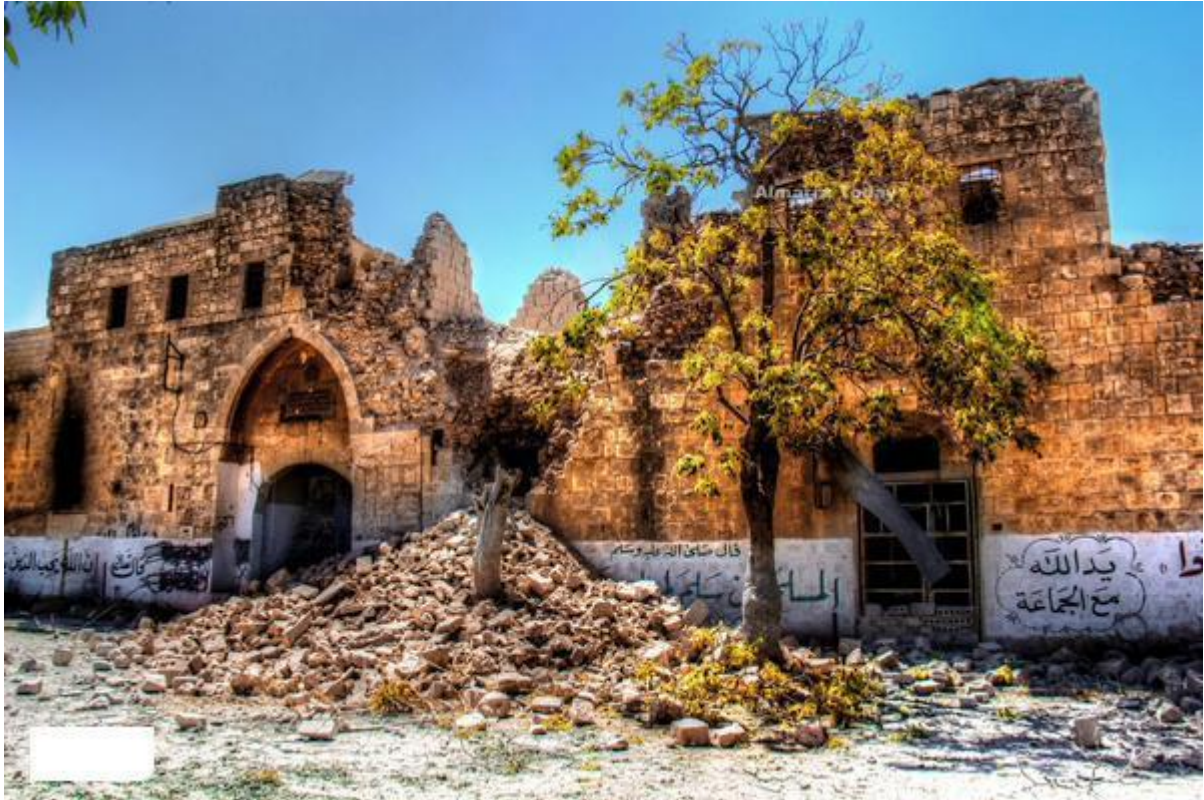
Khan Assad Pasha damaged (DGAM; August 10, 2015)
