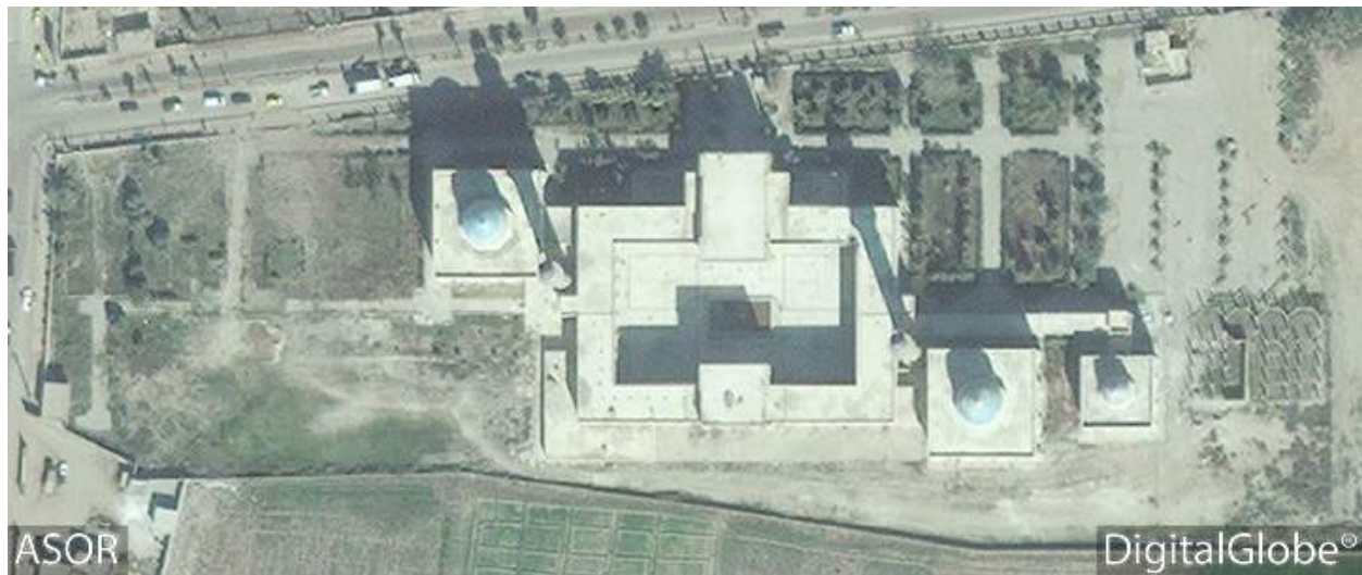
Shrine to Uwais al-Qurani and Ammar Bin Yasser, Raqqa, with no visible damage (DigitalGlobe; February 12, 2014)
